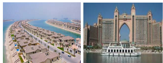
Fig. 14. Typical light weight and heavy structures in PJ
