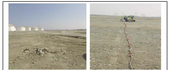
Fig. 27. Site photos showing leveling rockfill
