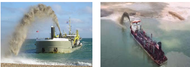
Fig. 4. Typical photos of sand dredging operations
